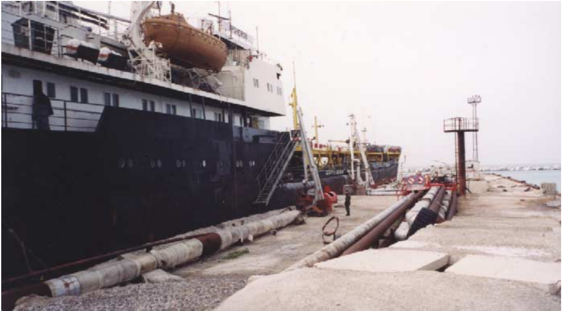
2. Tanker berthed alongside berth n°5 (notice poor piping system)
