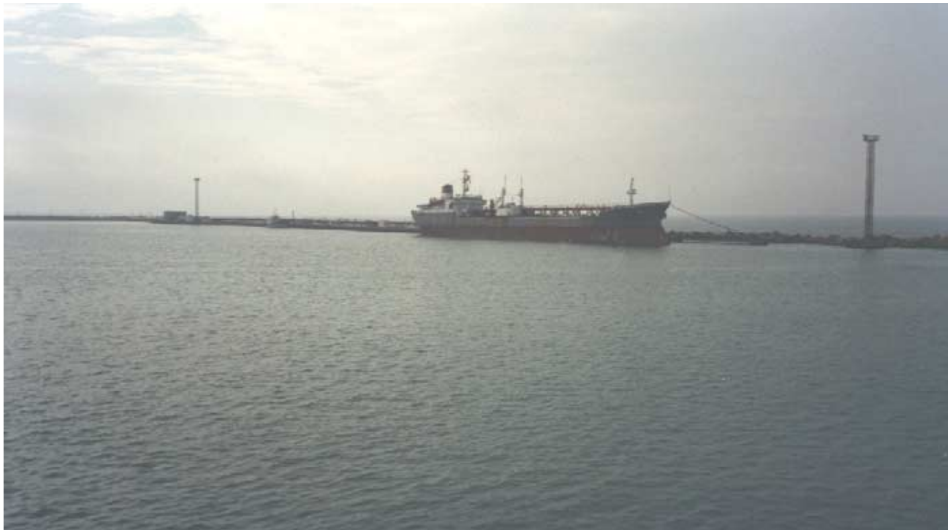
6. Berths n°9 and n°10 (notice low-crested breakwater)
